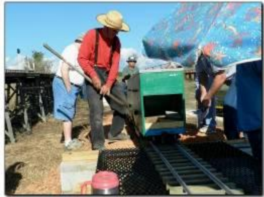
Bill Hays and John Bortz apply ballast with our new ballast car.
