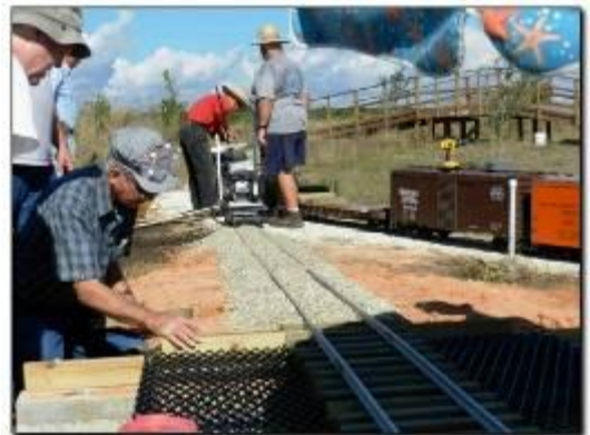
John Tribble installs track support. Behind Bill Hays runs power tamper.
